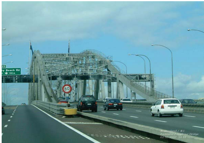
Auckland Harbour Bridge Moveable Median Barrier, Auckland, New Zealand
