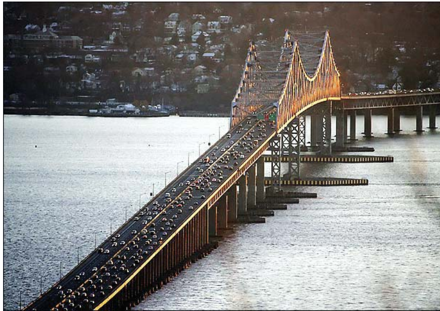
Tappan Zee Bridge Moveable Median Barrier, Tarrytown, NY
