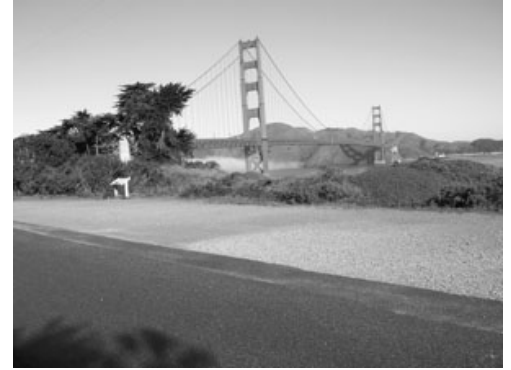
Exhibit 3-5 Battery East Road Turnout
