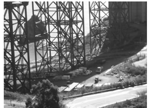
Exhibit 9-4 Northern Bridge Span Staging Area
