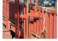
are then manually lifted over the outside handrail into place around a group of suspenders using a rope and pulley system. Workers enter the cable box after it is installed by climbing step ladders from the sidewalk level.
