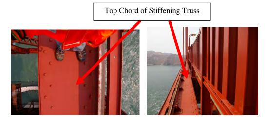
The maximum distance that personnel will have to walk along the truss top chord is 75 feet, since the gates are spaced 150 feet apart. The suspender ropes are spaced 50 feet apart, so there will be instances where workers will need to climb around the outside of the suspender ropes as they walk along the top chord to the travelers. There will also be instances where workers will need to climb around the belvederes on the traveler rail as discussed above.
