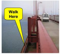
Fall protection will be required when walking from the gates to the travelers. It is proposed that a permanent stainless steel safety cable be installed on the outboard side of the east and west outside handrail or new barrier, along the entire length of the Bridge, for workers to "tie-off" to when walking along the stiffening truss upper chord or traveler rail. The cable will be on the outer face of the outside hand rail posts to minimize its visibility.
