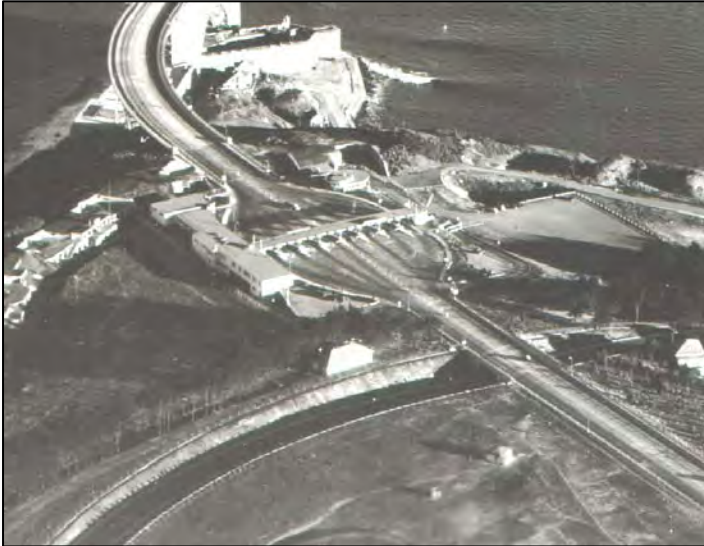
Figure 1. Detail of 1937 photograph showing Toll Plaza and bridge administration building, with west entrance to the Toll Plaza Undercrossing (34 0069) visible underneath the southern end of the building. (San Francisco History Center, San Francisco Public Library)
