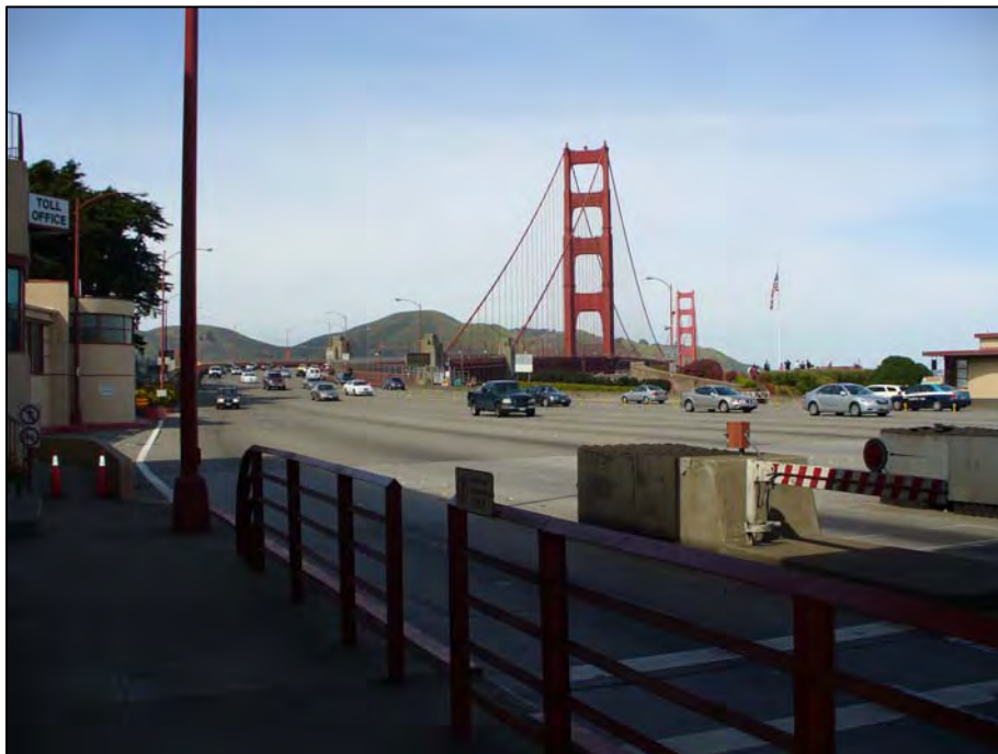
Photograph 9. Southbound lanes approaching Toll Plaza, view northeast, March 2007. [Source: JRP Historical Consulting, LLC]
