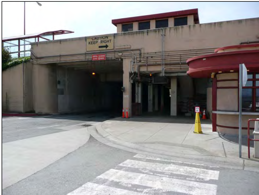
Photograph 11. East side of Toll Plaza Undercrossing (34 0069), view southwest, April 2008. [Source: JRP Historical Consulting, LLC]
