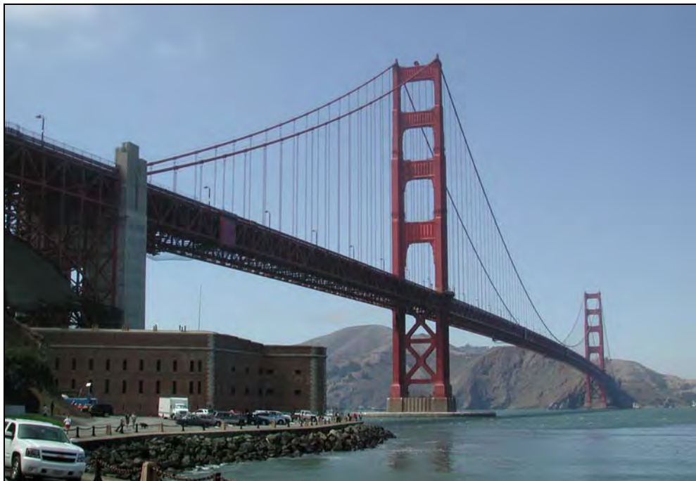
Photograph 2. View of east side of bridge from Fort Point, camera facing north, August 2007. [Source: MacDonald Architects]
