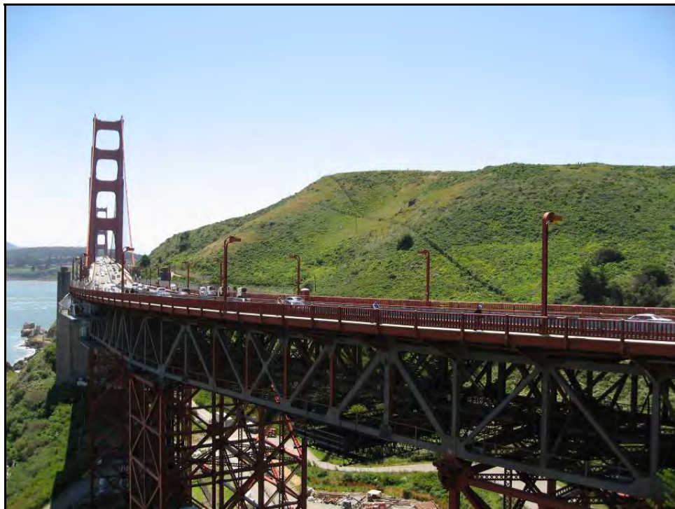
Plate 10. View from Vista Point, facing south (simulation)
