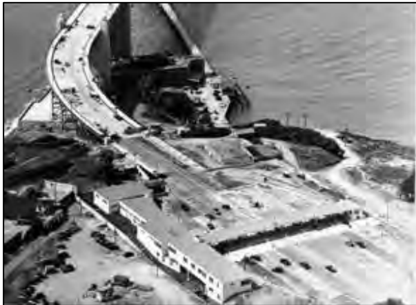
Plate 6. Detail of 1937 photograph showing Toll Plaza and Bridge Administration Building during Bridge construction, with west entrance to the Toll Plaza Undercrossing (34 0069) visible underneath the southern end of the building. (Permission pending: San Francisco Historical Photograph Collection, San Francisco Public Library)
