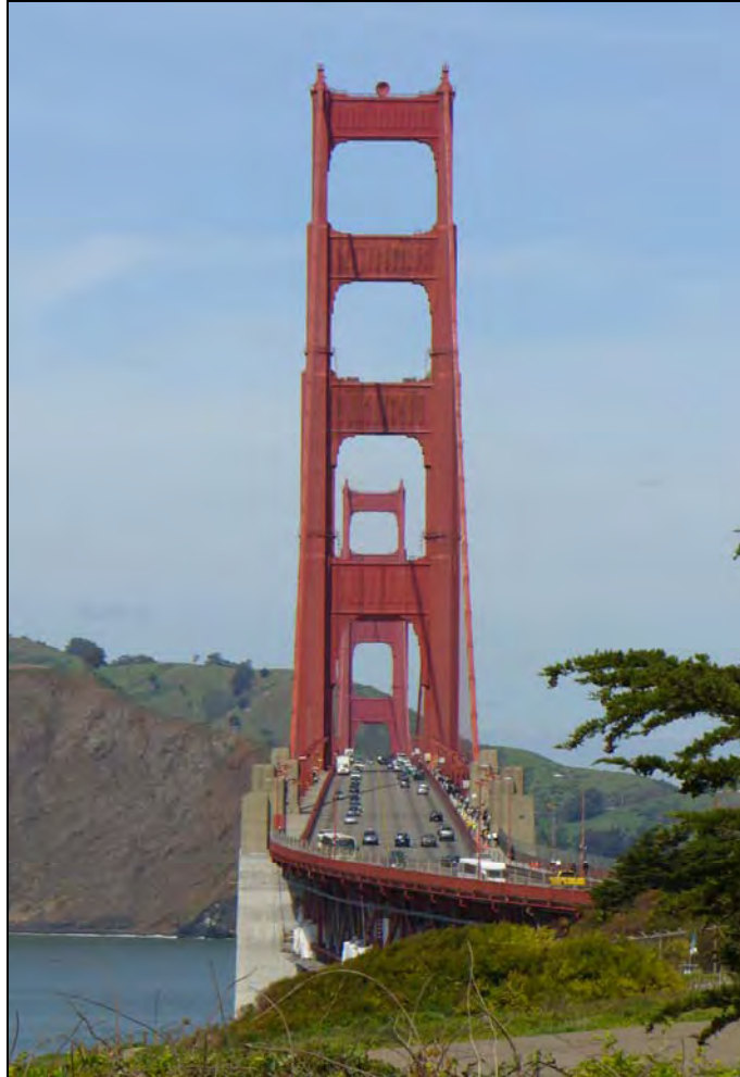
Photograph 5. View of bridge deck and towers (right), camera facing north, March 2007. [Source: JRP Historical Consulting, LLC]
