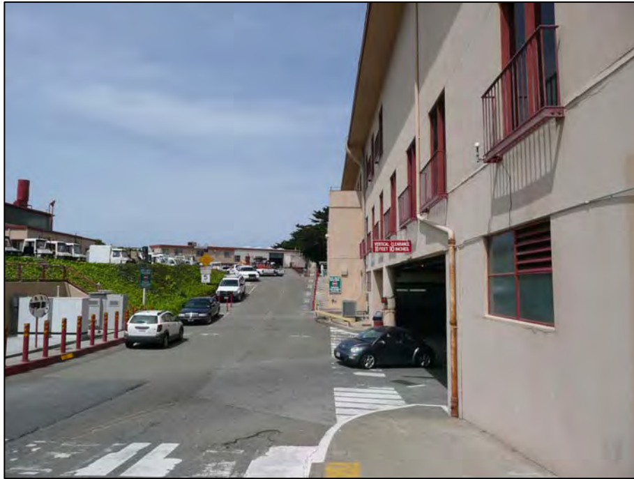
Photograph 10. West side of Toll Plaza Undercrossing (34 0069), view north, April 2008. [Source: JRP Historical Consulting, LLC]
