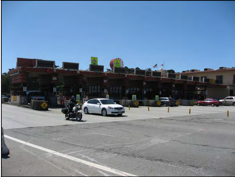
Plate 17. View of toll plaza from Round House Gift Center, facing south (existing)
