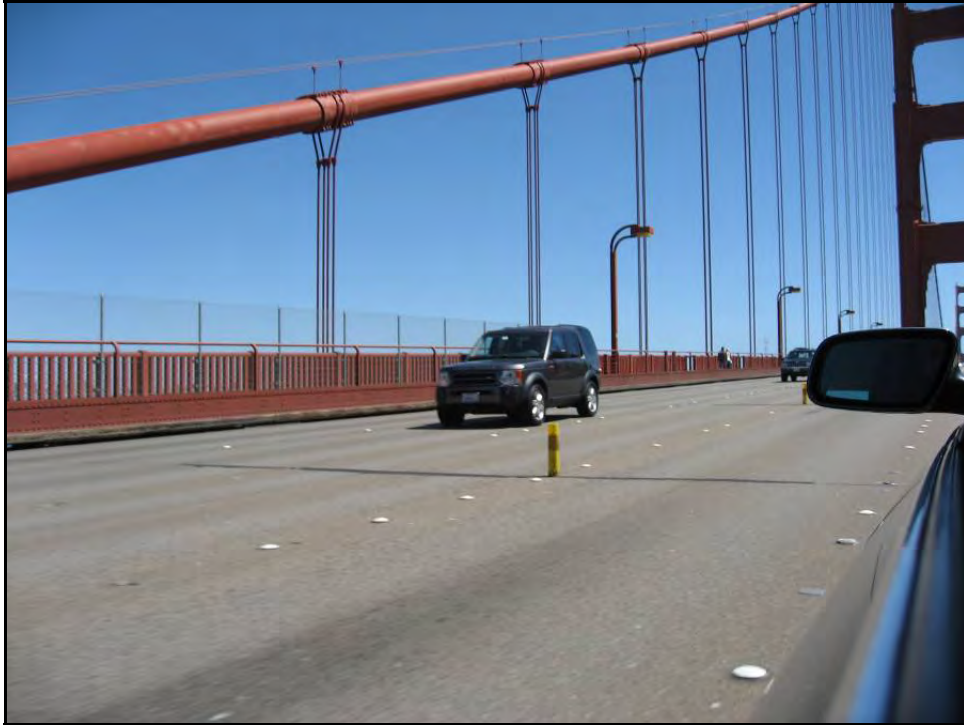
Plate 13. View while driving across Bridge, facing southeast (existing)
