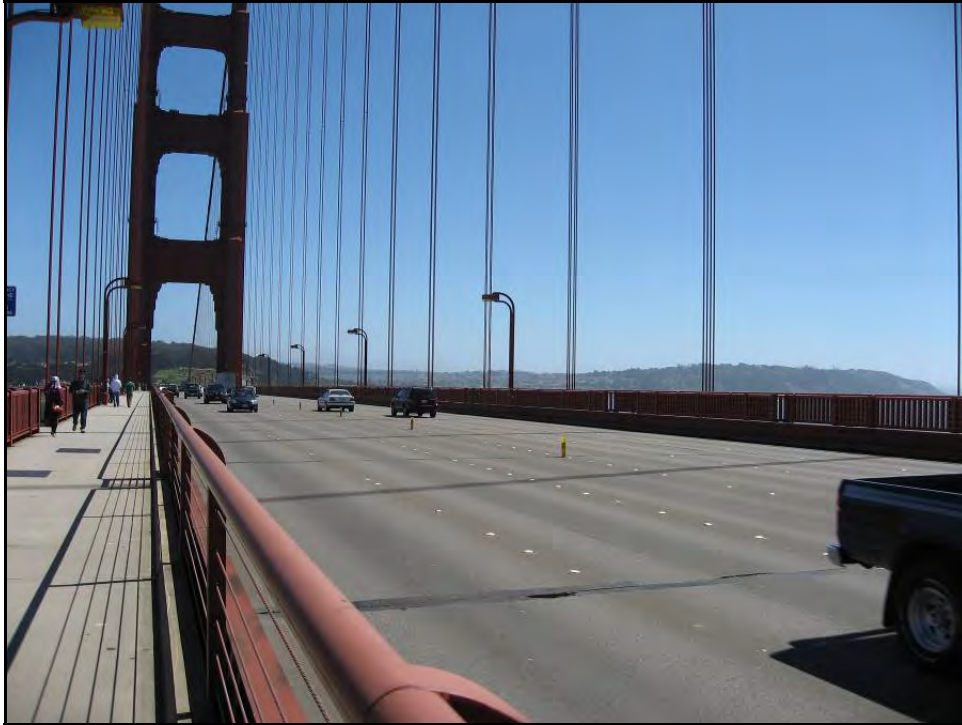
Plate 11. View from pedestrian walkway along Bridge, facing southwest (existing)
