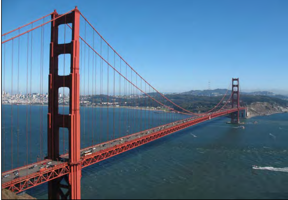
Photograph 1. View of west side of bridge, camera facing south, August 2007. [Source: MacDonald Architects]
