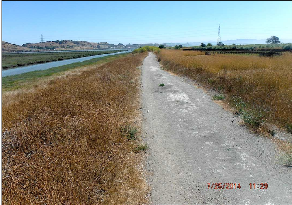
Figure 22. View of the modern levee road at northern edge of the ADI, facing east (July 24, 2014).
