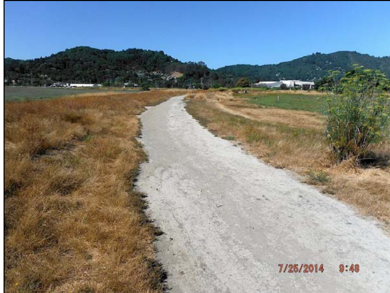
View of the levee road at the ADI's southern end, facing southwest (July 24, 2014).
