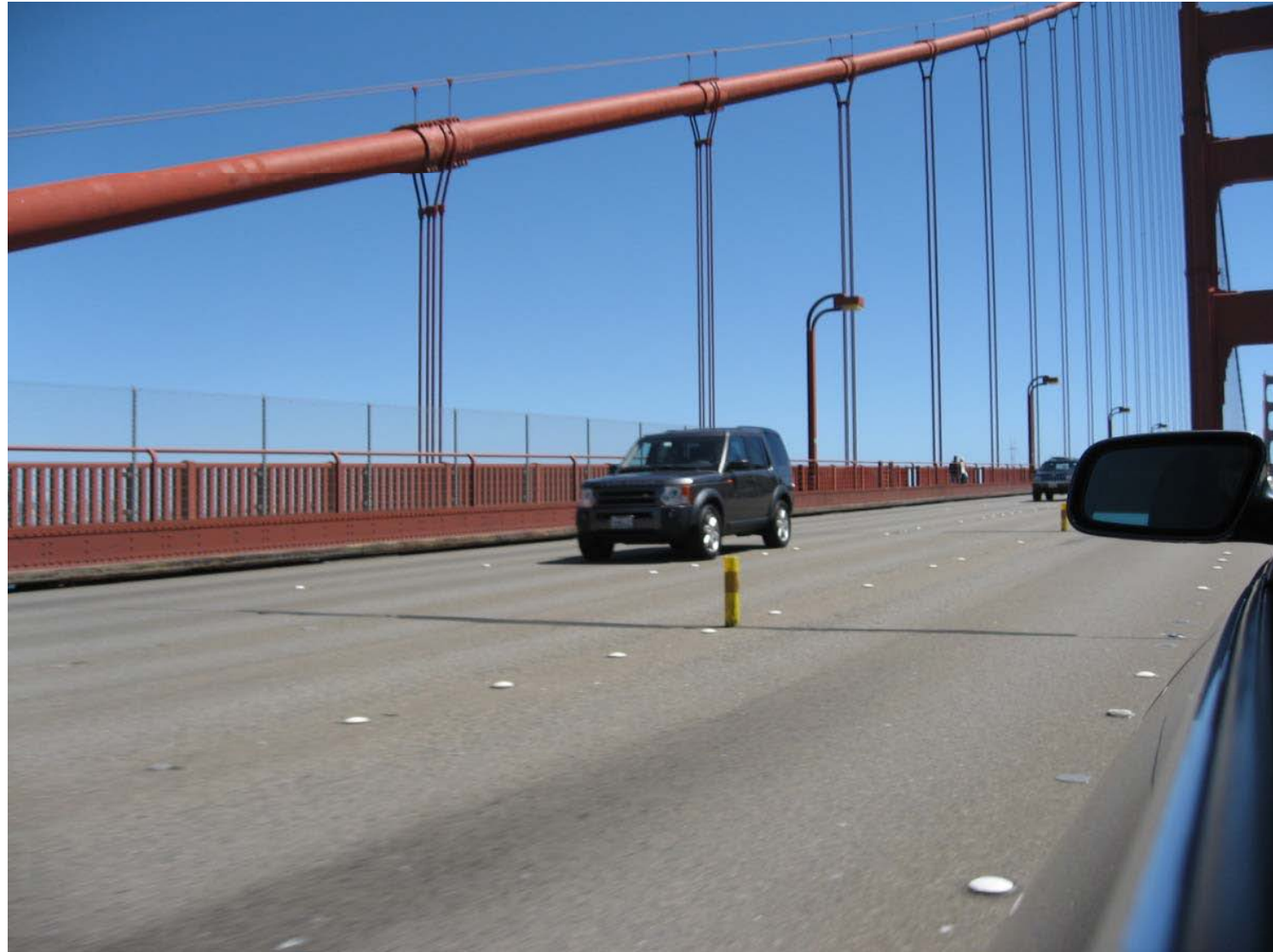
KOP 7, Driving South Across Bridge Looking Southeast (Existing)
