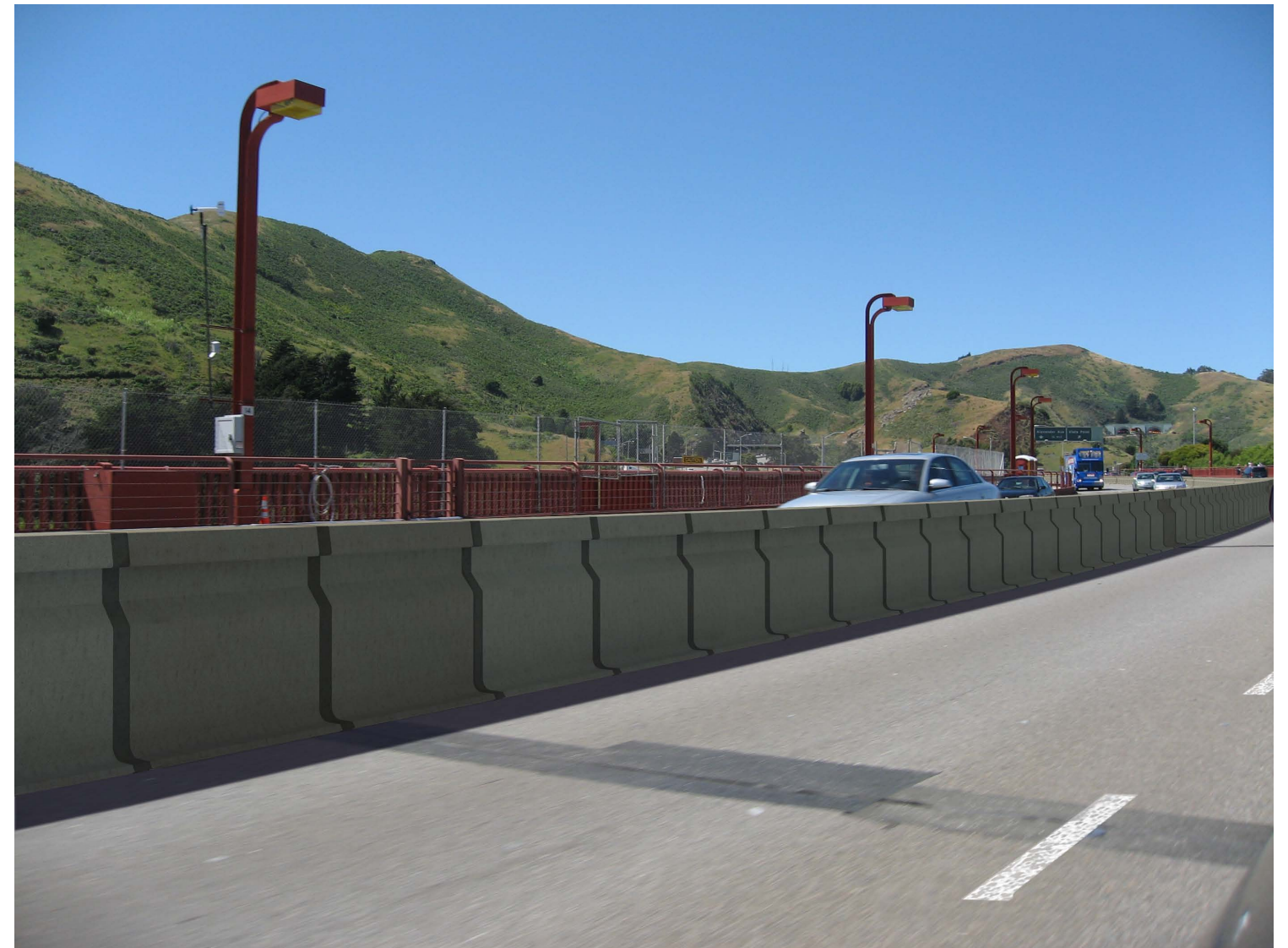
KOP 8, Driving North Across Bridge Looking Northwest (Simulation)
