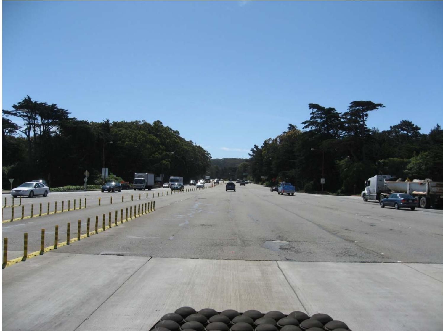
KOP 2: Toll Plaza Looking Southeastt (Existing)
