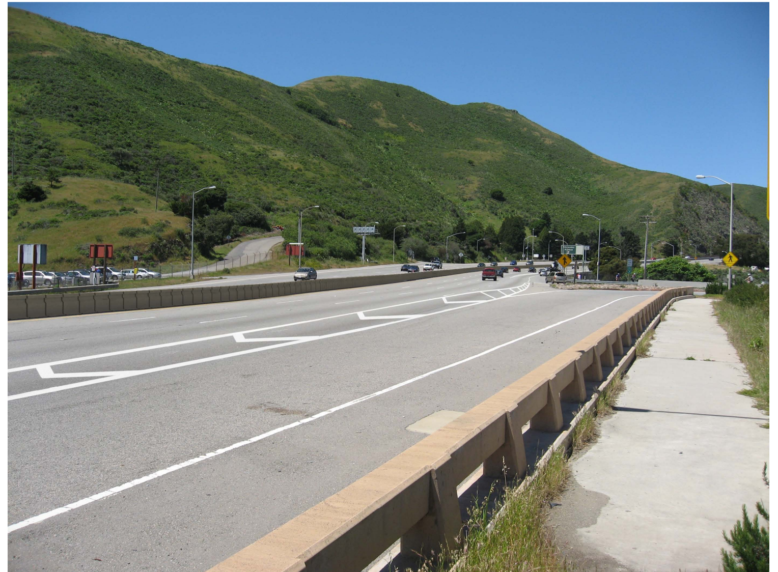
KOP 10, Bicycle Trail Near Vista Point Looking Northwest (Simulation)
