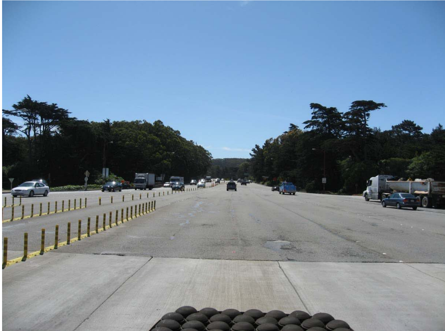
KOP 2: Toll Plaza Looking Southeast (Existing)
