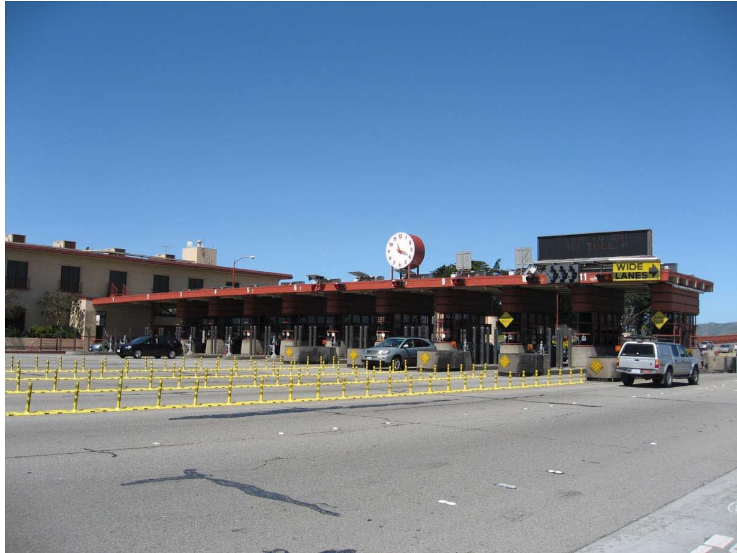
KOP 4, Bus Stop at Toll Plaza Looking Northwest(Existing)
