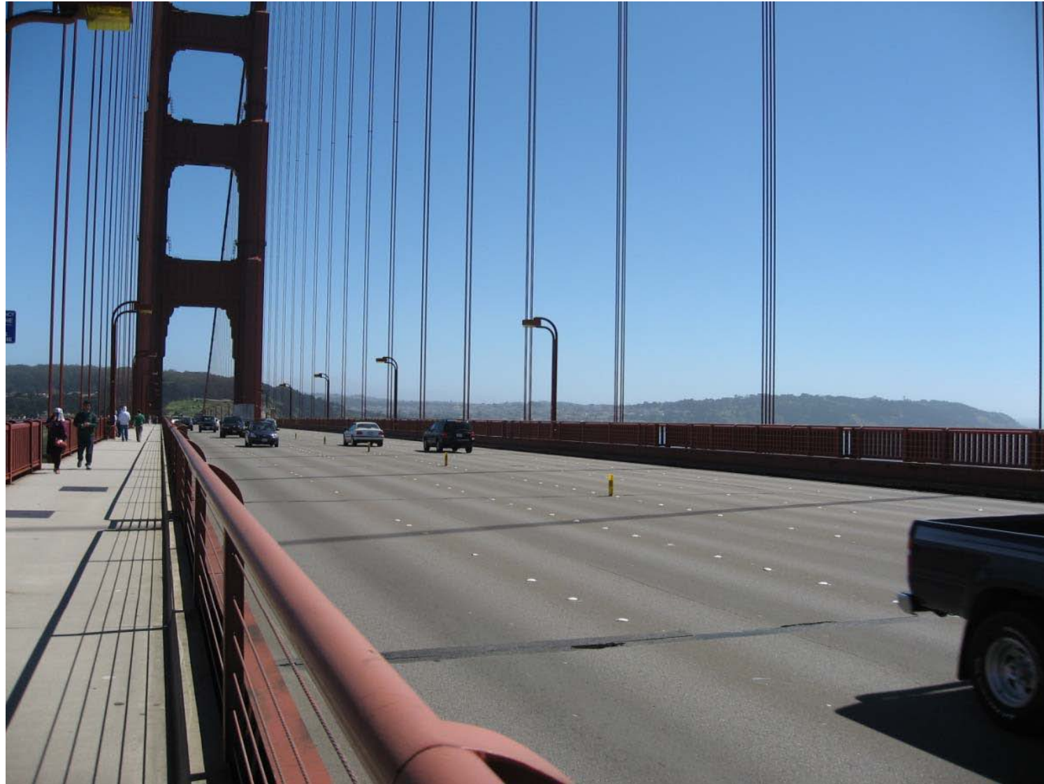
KOP 5, Pedestrian Walkway Along Bridge Looking Southwest (Existing)
