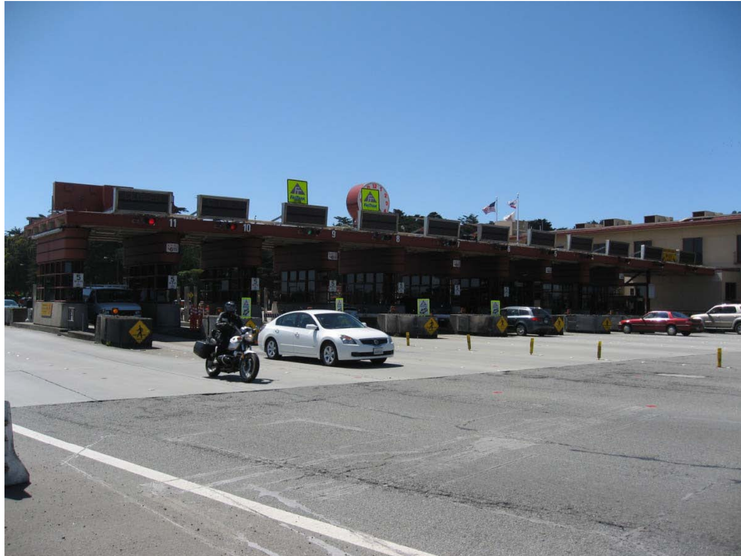
KOP 3: Bridge Gift Center Looking South (Existing)
