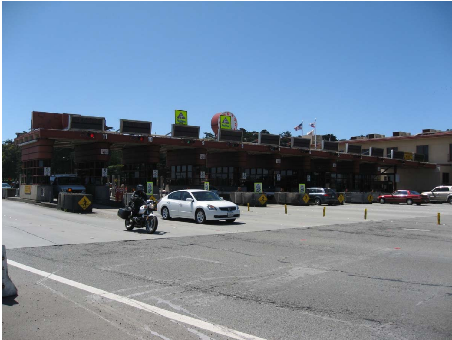
KOP 3: Bridge Gift Center Looking South (Existing)
